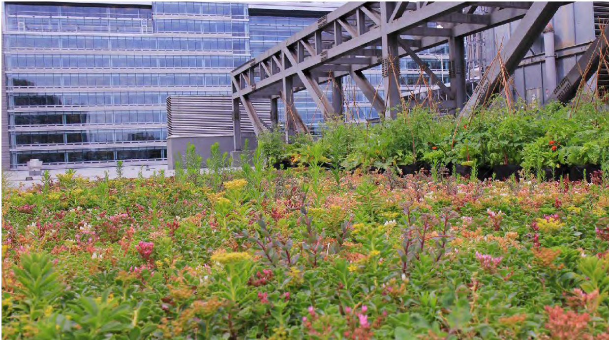
Green Roof Supporting Urban Biodiversity
