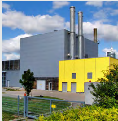
Central Heating Plant, Germany
