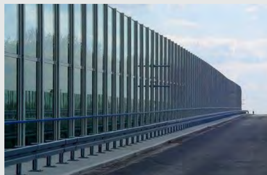
Sound Barrier Wall with High Quality Architecture, Gaschwitz, Germany
