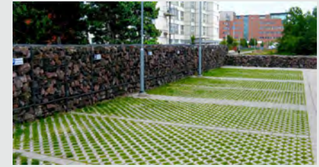
Permeable Parking Surface, Stockholm, Sweden
