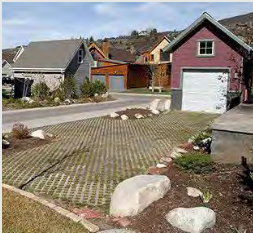
Pervious Parking Surfaces
