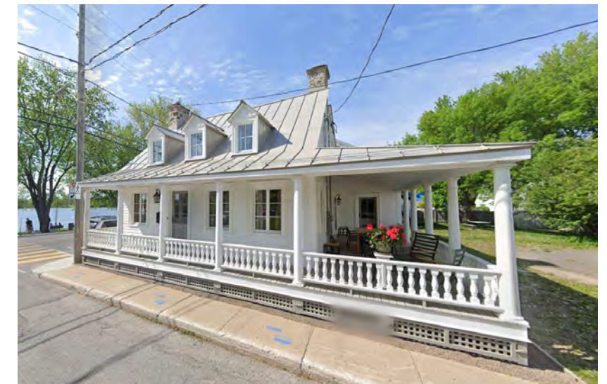
FIGURE 104. PROPER INTEGRATION OF RENOVATION (AFTER)
