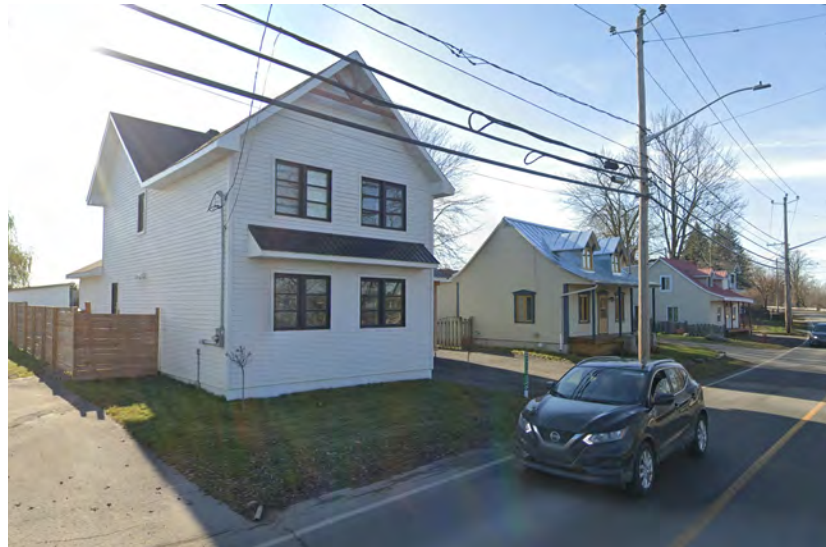
FIGURE 131. INADEQUATE INTEGRATION OF NEW CONSTRUCTION
