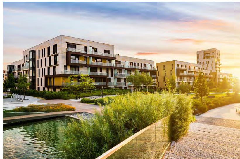
FIGURE 76. VANNES PERION ECO-DISTRICT
