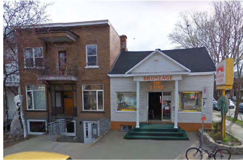
FIGURE 99. INADEQUATE INTEGRATION OF A NEW CONSTRUCTION (BEFORE)
