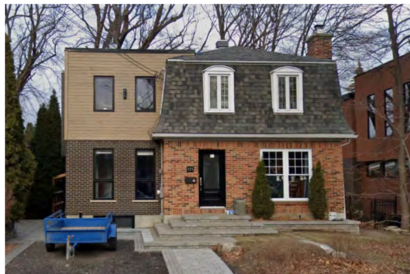
FIGURE 134. INADEQUATE INTEGRATION OF AN EXPANSION
