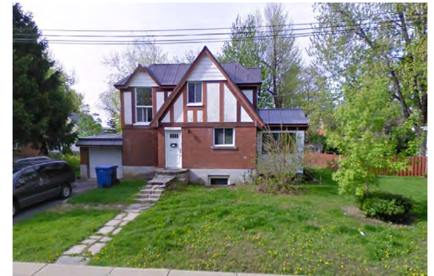
FIGURE 135. INADEQUATE INTEGRATION OF RENOVATION (BEFORE)
