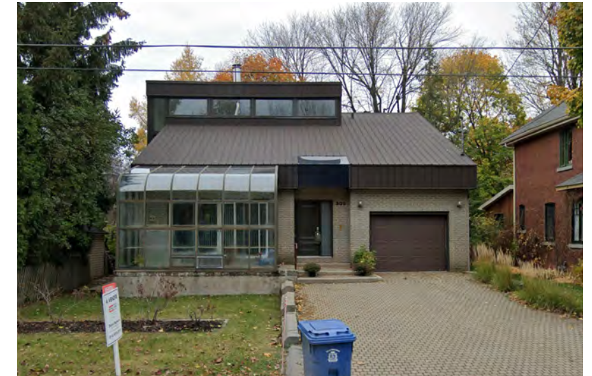
FIGURE 16. PROPER INTEGRATION OF RENOVATION (BEFORE)
