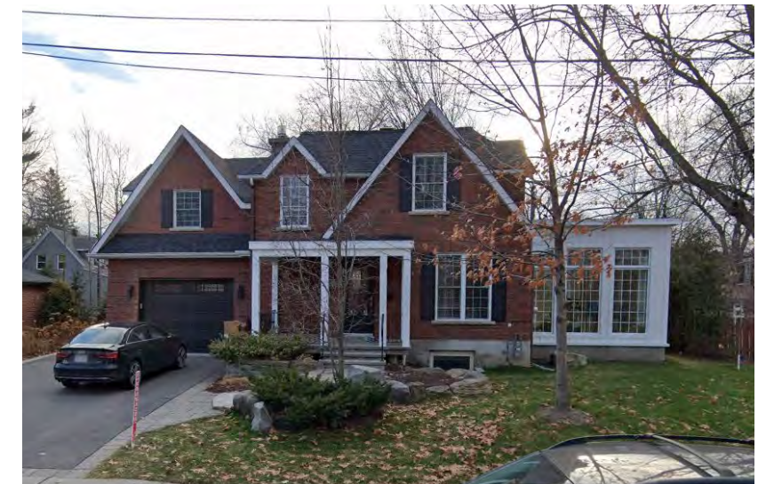
FIGURE 136. INADEQUATE INTEGRATION OF RENOVATION (AFTER)
