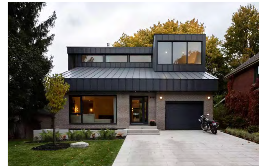
FIGURE 17. PROPER INTEGRATION OF RENOVATION (AFTER)
