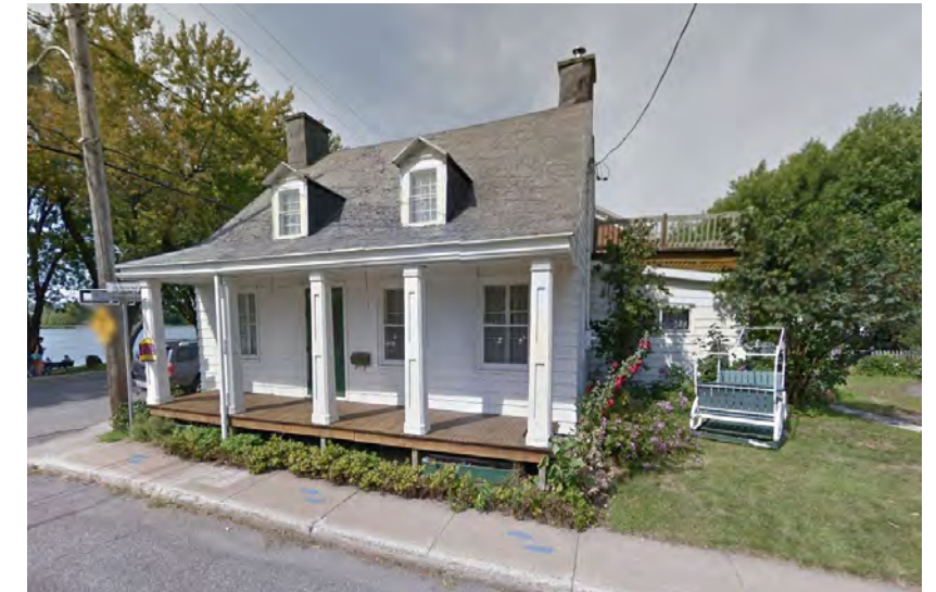
FIGURE 103. PROPER INTEGRATION OF RENOVATION (BEFORE)
